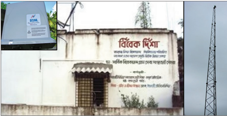
Figure 2. The education and healthcare center equipped with our WiMAX-based last-mile telecommunication solution. The figure on the right shows the mast used to host the WiMAX CPE, and the inset shows the WiMAX CPE that connects to the base station [1].
